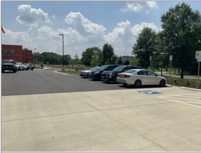
OVERVIEW OF ACCESSIBLE PARKING AREA
