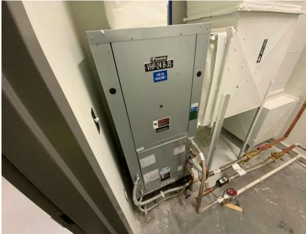
25 - WATER SOURCE HEAT PUMP
