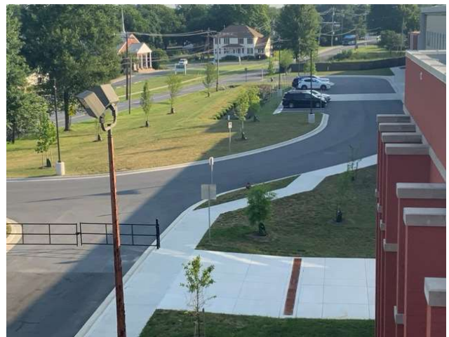
28 - SECONDARY PARKING AREA
